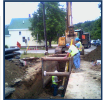
Contractors install water main on Churchill Street during a 2008 District project
